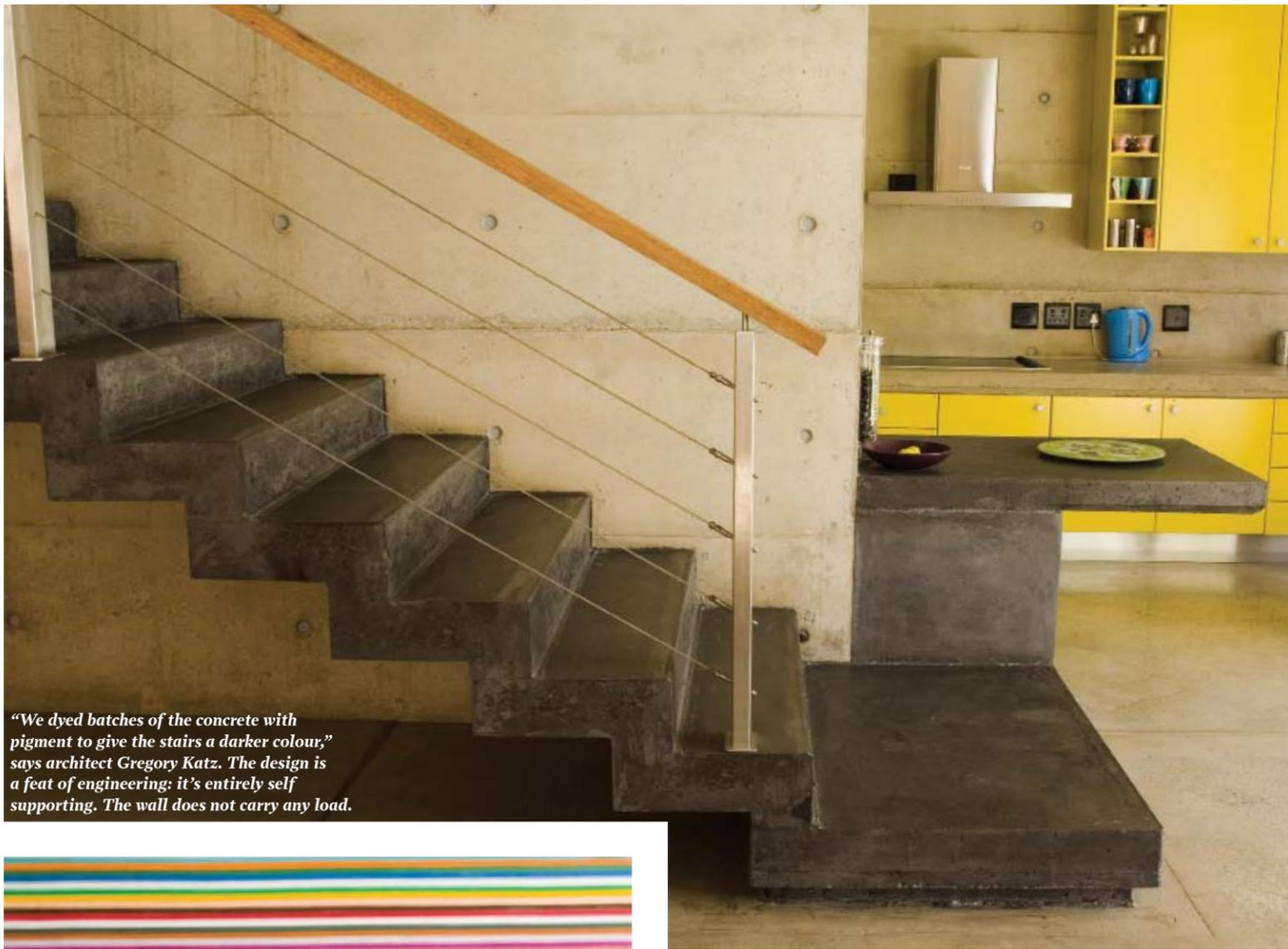
*"We dyed batches of the concrete with pigment to give the stairs a darker colour," says architect Gregory Katz. The design is a feat of engineering: it's entirely self supporting. The wall does not carry any load.*
